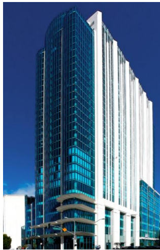
Double pane insulated w/ low-e
