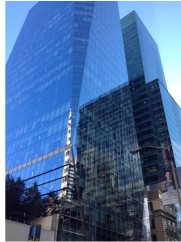
Double pane insulated w/ low-e
