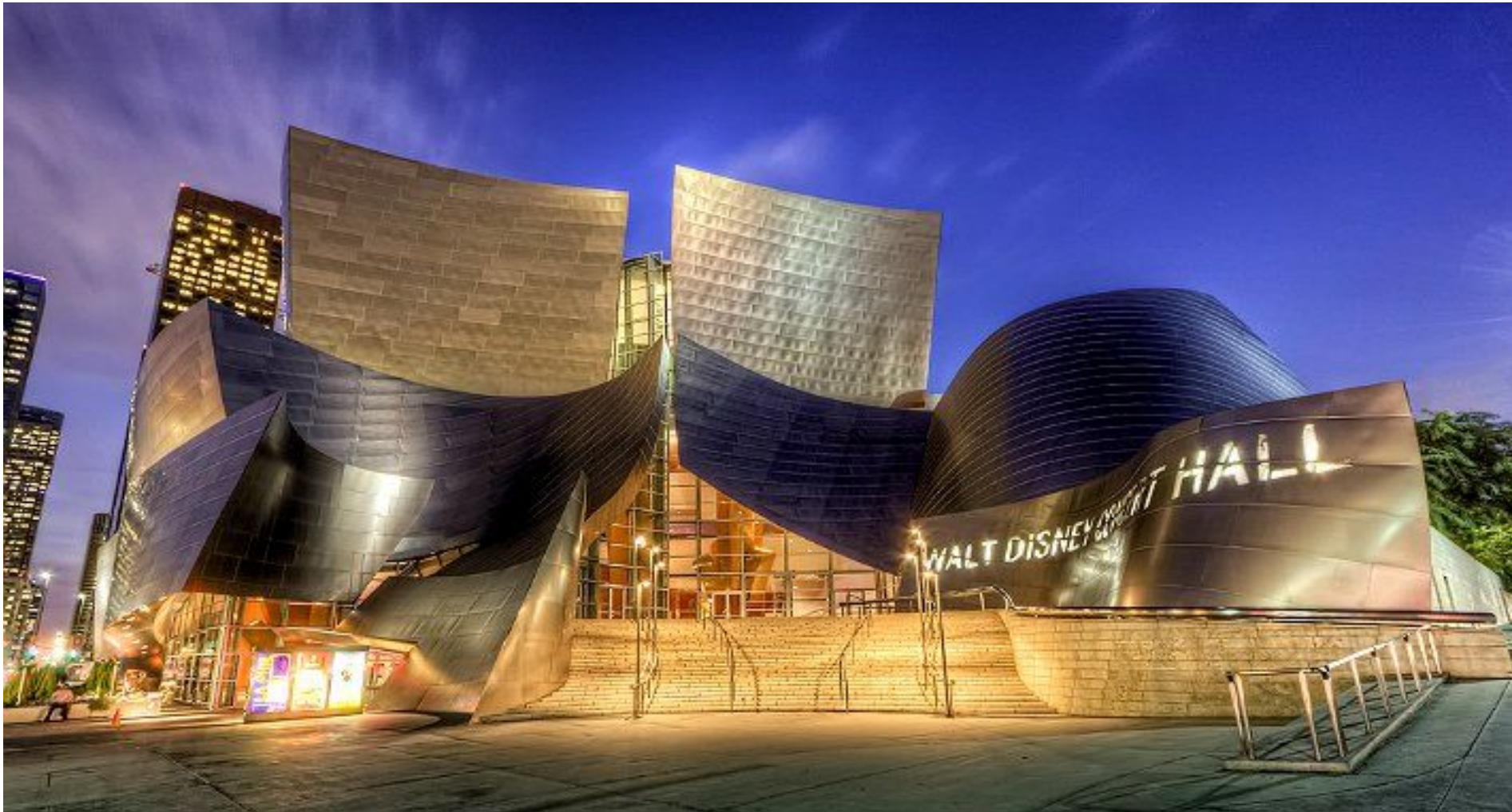
Walt Disney Concert Hall - Los Angeles, CA Gehry Partners
