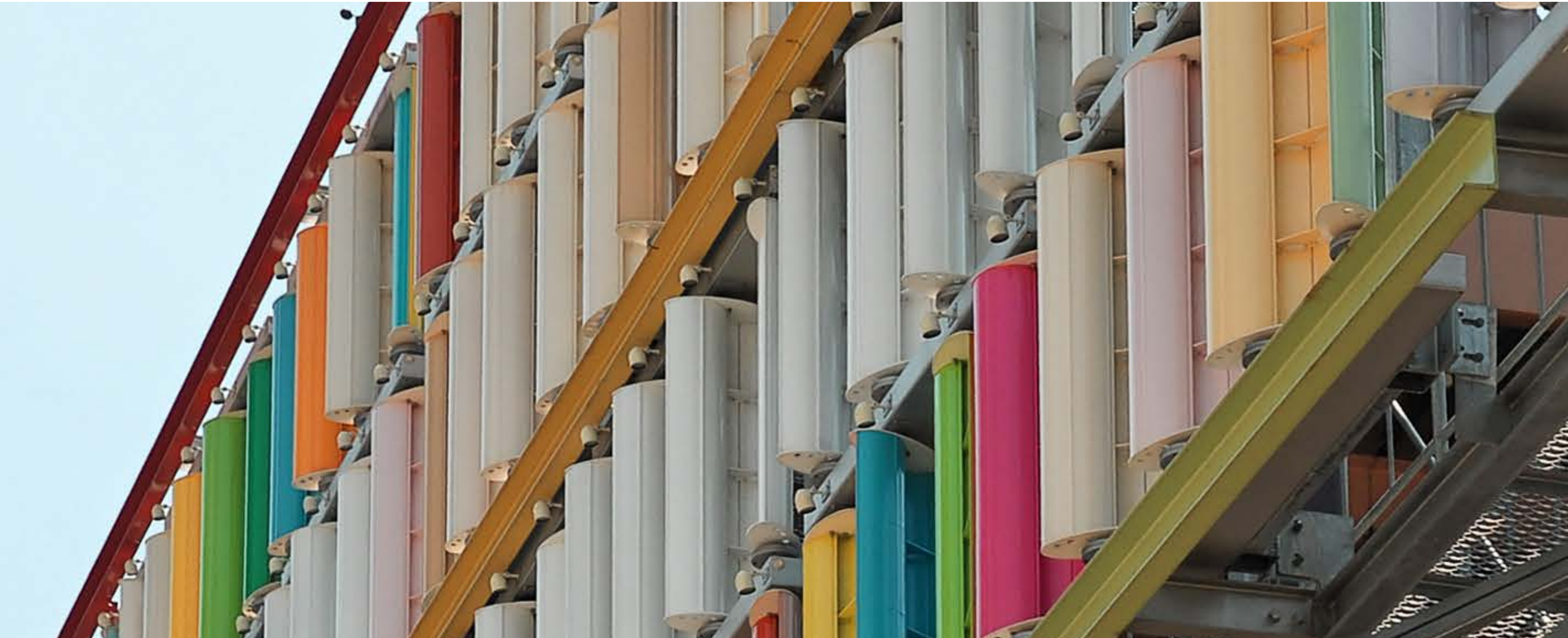
Inaba Electric Works, Eco-Curtain, Nagoya, Japan, 2005
