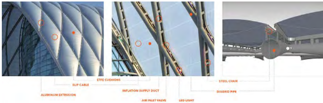
1. STRUCTURAL DESIGN OF ETFE ROOF REDUCES STEEL TONNAGE
