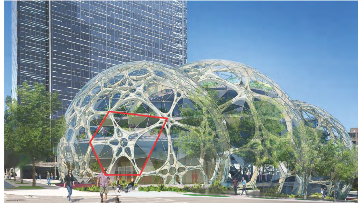
Structural Steel Catalan Module
