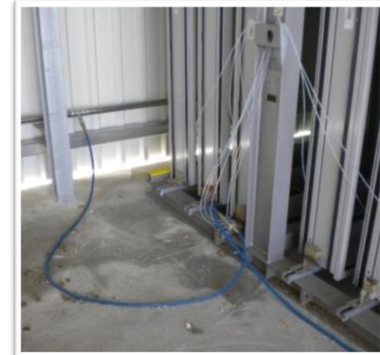
Security of cavity condition in storage
