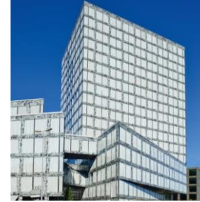
Richti-Areal Baufeld 1, 7, Wallisellen
