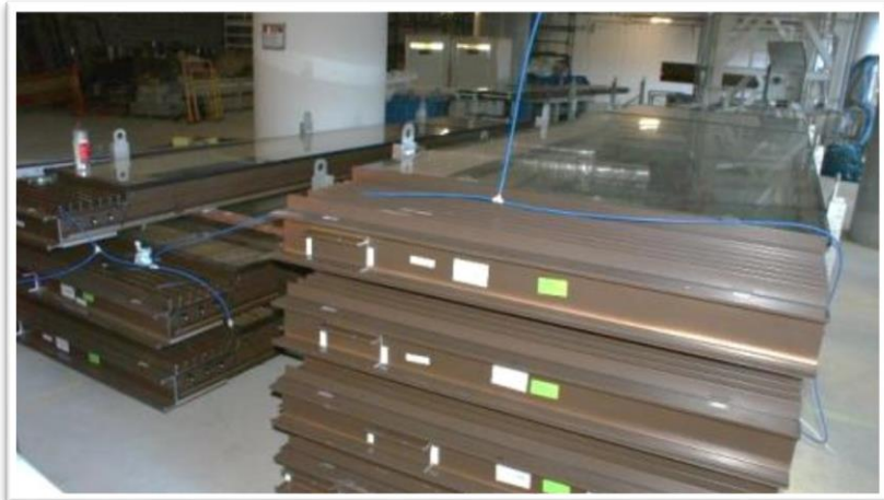
Security of cavity condition during pre-installation on site
