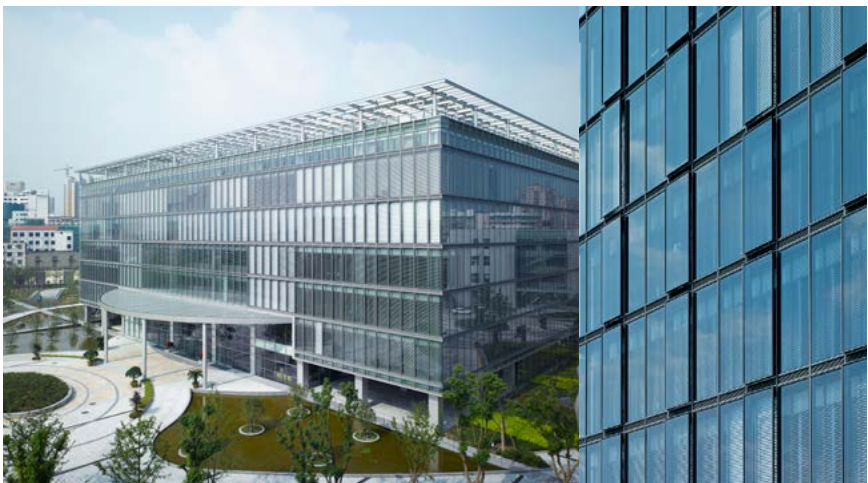
FIG. 1: DYNAMIC DOUBLE-SKIN FACADE AS PART OF A COGNITIVE BUILDING CONCEPT (SHANGHAI TOBACCO BUILDING, CN-SHANGHAI (2005), HUANG FANG / SHANGHAI PAN-PACIFIC ARCHITECTURAL DESIGN CO. LTD.).
