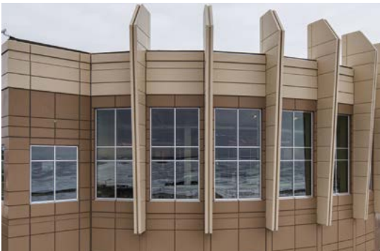
FIG. 3B: GENERATION 2 EC GLASS WITH IMPROVED BLUE/GREEN EXTERIOR AESTHETIC, MORE TYPICAL OF LOW-E GLASS PRODUCT.
