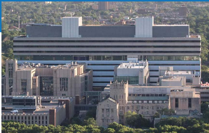
UNIVERSITY OF CHICAGO MEDICINE - CENTER FOR CARE AND DISCOVERY. IMAGE © TOM ROSSITER, COURTESY OF RAFAEL VIÑOLY ARCHITECTS
