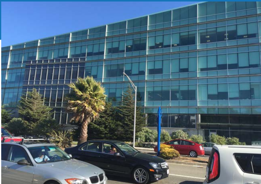
FIG. 1: WHILE MANUAL BLINDS ARE USED TO CONTROL GLARE, THEY ARE OFTEN LEFT DRAWN LONG AFTER THE GLARE CONDITION HAS PASSED, NEGATING THE BENEFITS OF DAYLIGHT AND VIEW.
