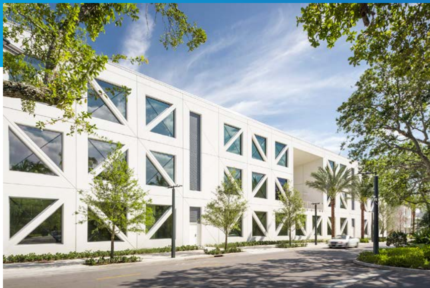
FIG. 6: A LARGE-SCALE INSTALLATION OF TRIANGULAR-SHAPED EC GLAZING AT THE FROST SCHOOL OF MUSIC IN MIAMI. NOTE THE ARCHITECTURALLY FAVOURED BLUE EXTERIOR REFLECTED COLOR. PHOTO COURTESY OF MORIS MORENO.
