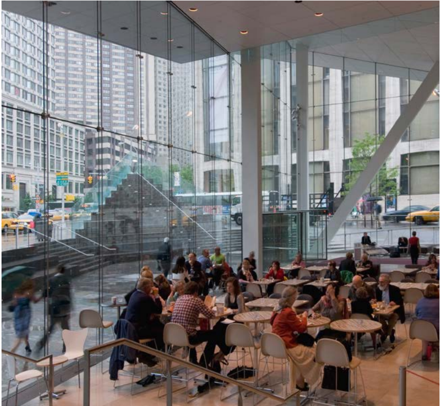
THE ALICE TULLY HALL RENOVATION BY DILLER SCOFIDIO + RENFRO AND FXFOWLE IN NEW YORK CITY FEATURES A ONE-WAY CABLE NET STRUCTURE SUPPORTING OVERSIZED GLASS PANELS WITH AN IONOPLAST INTERLAYER.
