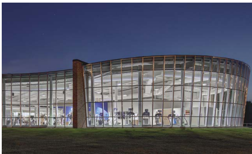
FIG. 5: A LARGE-SCALE INSTALLATION OF EC GLAZING AT BUTLER COUNTY HEALTH CARE CENTER IN DAVID CITY, NEBRASKA. THE APPLICATION FEATURES A COMPLEX CURVED FACADE WITH GLAZING SLOPED OUTWARDS. THE ARCHITECTS CHOSE EC GLAZING BECAUSE OF ITS ABILITY TO CONTROL HEAT AND LIGHT, AND ITS ABILITY TO MAINTAIN VIEWS OF NATURE FOR PATIENTS IN THE REHABILITATION CENTER. PHOTO COURTESY OF DAUBMAN PHOTOGRAPHY.
