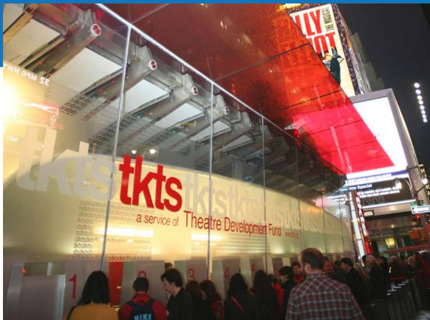
THE TKTS BOOTH BY PERKINS EASTMAN IN NEW YORK CITY WAS THE LARGEST LOAD-BEARING GLASS STRUCTURE IN THE WORLD AT THE TIME OF ITS COMPLETION. IT FEATURES AN IONOPLAST INTERLAYER FOR STRUCTURAL ENHANCEMENTS. 1
