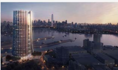
View of a proposed Brooklyn high-rise sheathed in HOK's Circadian Curtain Wall concept
